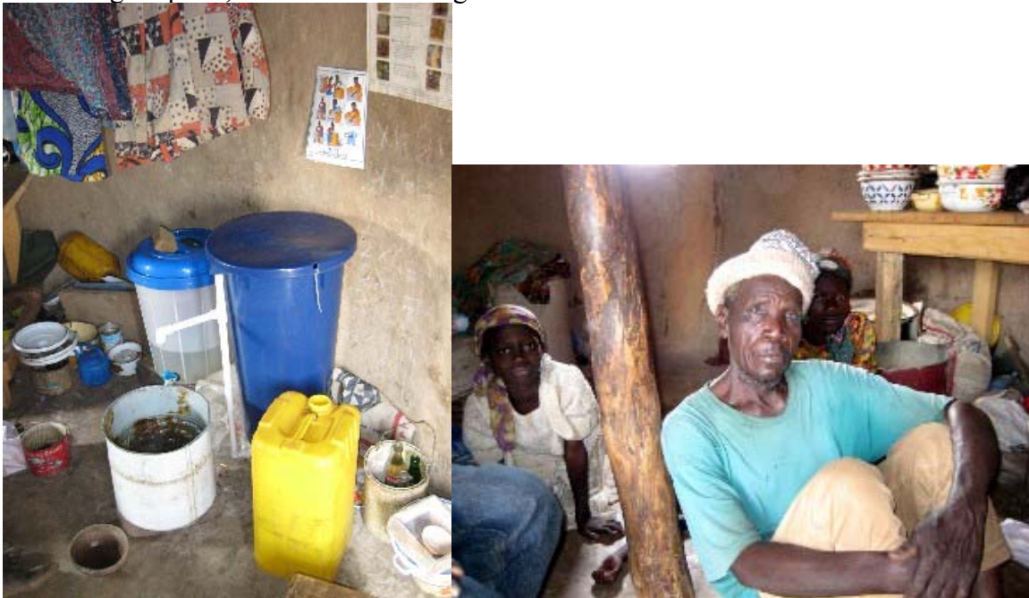
(1) Suliemana’s Kosim , BSF, metal BSF storage, and fetching jerrycan. BSF storage practices are not ideal (uncovered rusty drum). Note the BSF training material shown. (2) Suliemana and his daughter during interview
